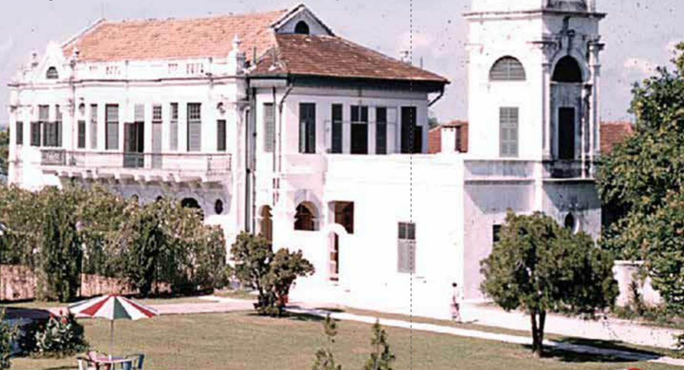
(Facing page) A rare colour photo of The Grand Hotel with its striking tower (building No. 26) taken by an unknown serviceman from RAF Changi before land reclamation works began, c. 1958. The round fountain pavilion where Moona Kader Sultan received his Legion d'Honneur is seen on the left. Courtesy of RAF Changi Association.
