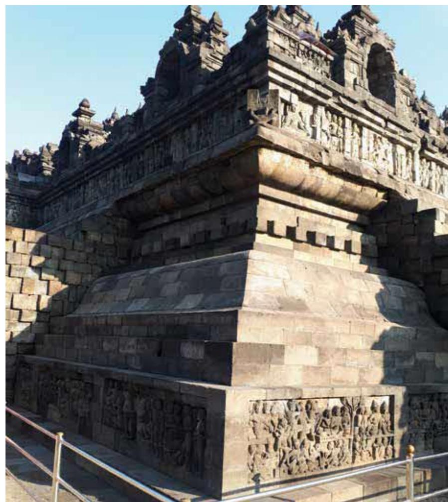
The four previously hidden panels located at the base of the southeastern corner of Borobudur, 2017. Photo by Erni Salleh.
